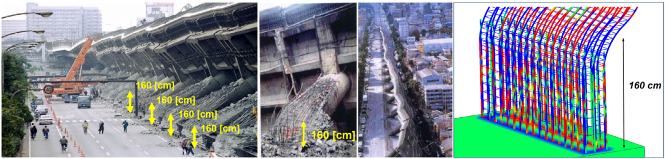
FIGURE 22 Destruction of viaduct supports of the Hanshin route (Kobe, 1995)
