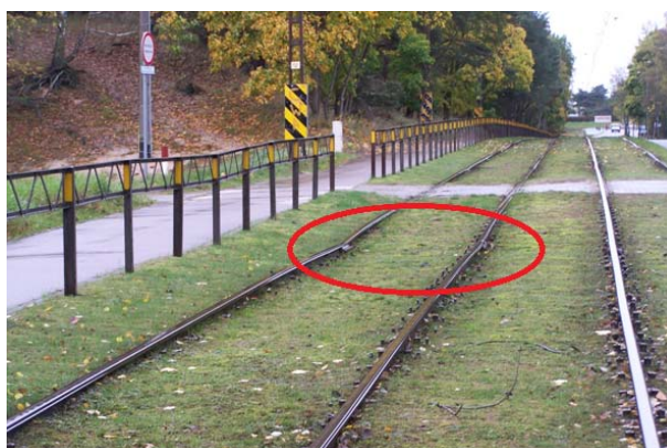
Fig. 3. Displacements of the sleepers in the track
