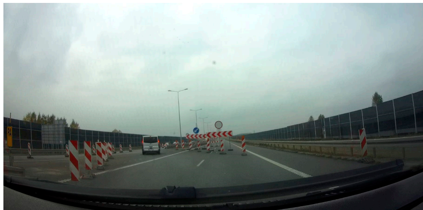
Figure 5. Example of a recorded event—unexpected road works.
