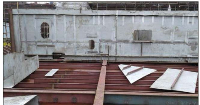
Fig. 1. RSW cargo tank under construction in shipyard
