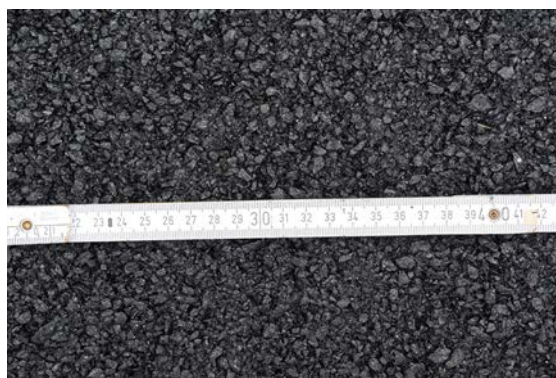
Figure 12. Finished texture of the poroelastic wearing course.
