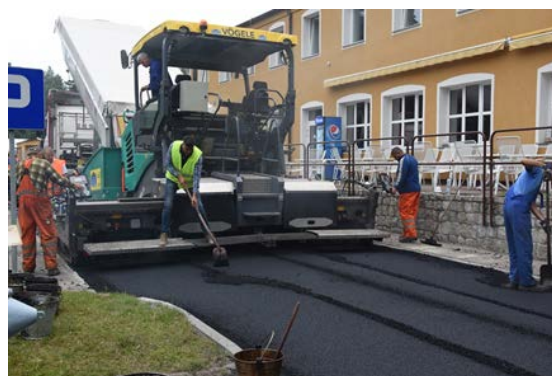
Figure 11. Paving of the poroelastic mixture.
