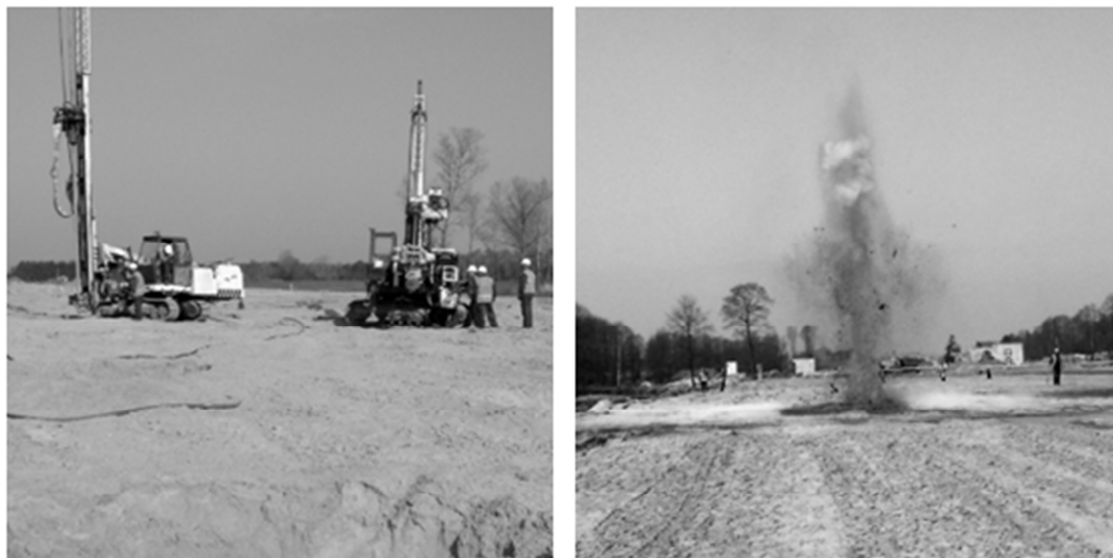
10. The method of subsoil improvement using blasting agents, A2 motorway, Koło-Dąbie section [9]
