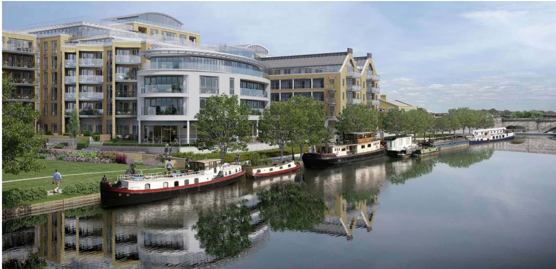
Fig. 1. Narrowboats moored next to Kew Bridge in London. Source: www.berkeleygroup.co.uk.
