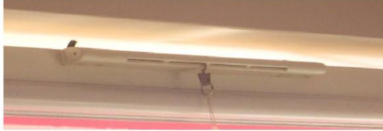
Fig. 2. Typical inlet gaps in Poland
