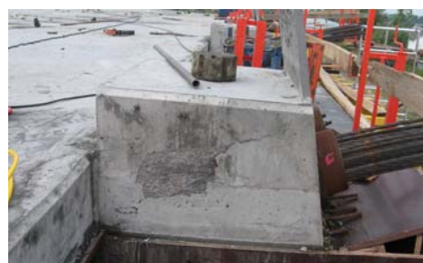
Fig. 3. Damaged cantilever no. 4 after prestressing
