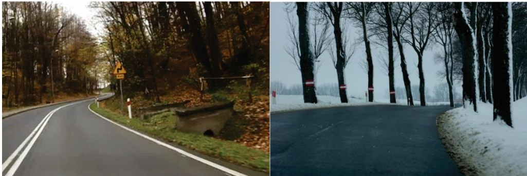
Fig. 1 Examples of roadside hazards on horizontal curves.
