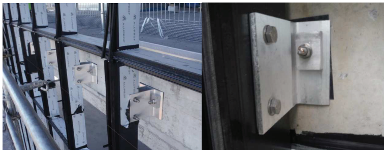
Fig. 1. Mullion-transom wall system – aluminium profiles and brackets
