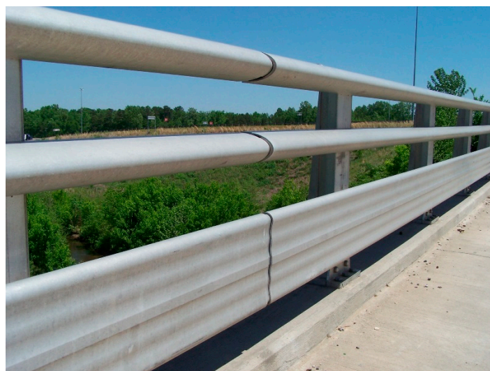
Figure 1. A three-bar metal bridge rail [1].
