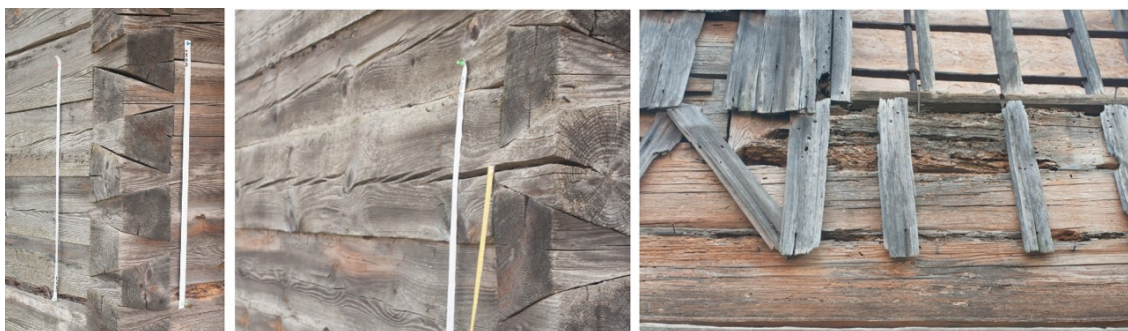
Figure 6. The church in Cewków: wall corner, longitudinal cracks in the wall, visible cavities in the wall.
