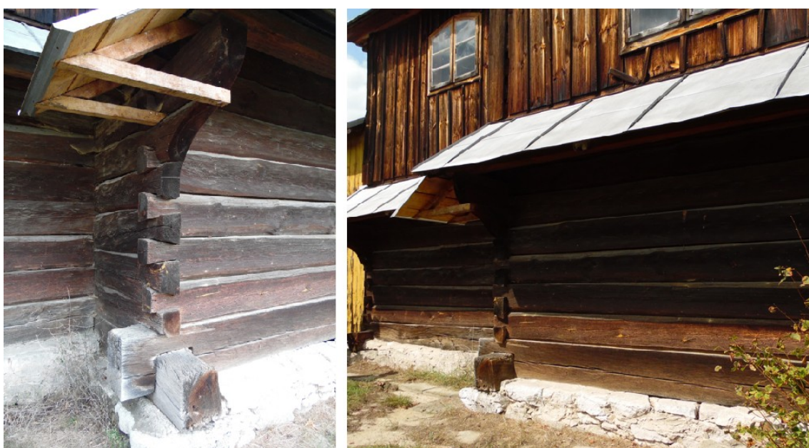
Figure 10. Current condition of log walls with dovetail notches in Chotylub: cracks in log walls in and contemporary repairs of the eaves roof.
