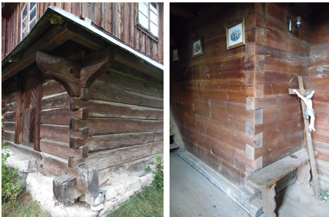
Figure 9. Current condition of log walls with dovetail notches in Chotylub outside and inside.
