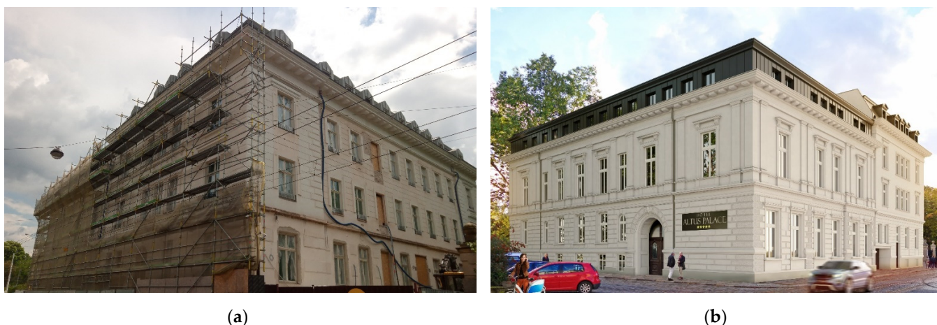
Figure 1. Former Leipziger Palace in Wrocław: (a) view on the facade during reconstruction; (b) facade visualization after reconstruction to the hotel building.
