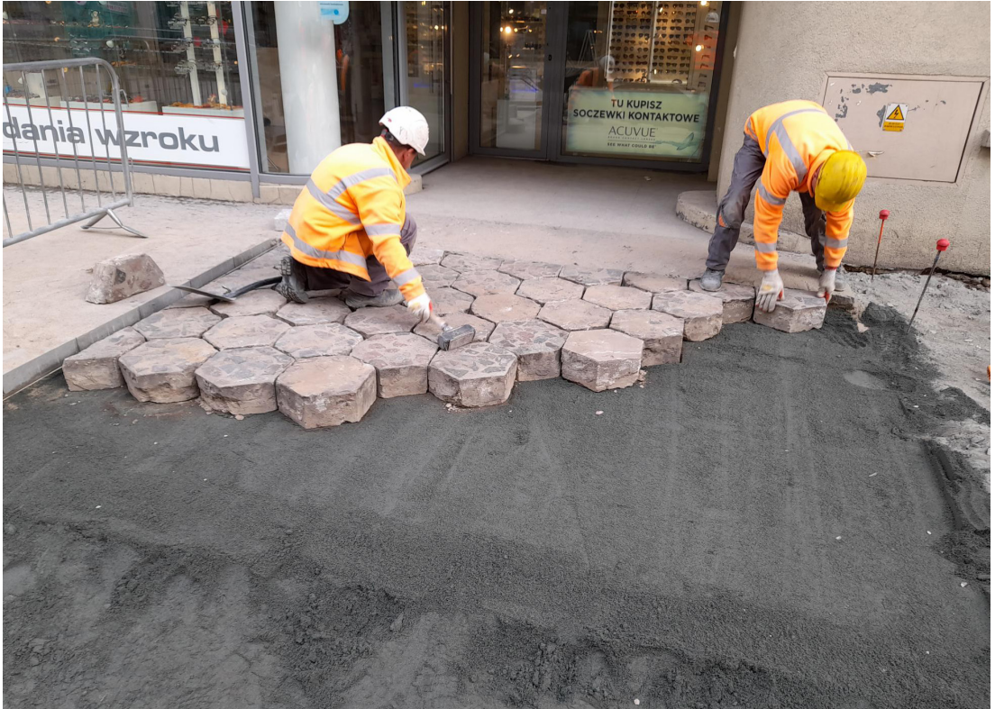
Fig. 4. Gdynia, Starowiejska Street during renovation works in 2022, which involved relocating the historic surface made of hexagonal blocks; photo by R. Hirsch.
