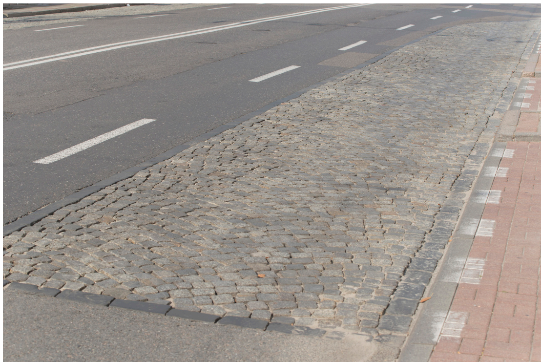
Fig. 2. Gdynia, 10 Lutego Street, historic road surface at the turn of the 1920s and 1930s, where asphalt was combined with cobbled side lanes; photo by B. Ponikiewski.
