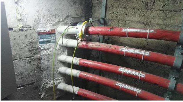
Fig. 6. Inductive couplers installed at point B.
