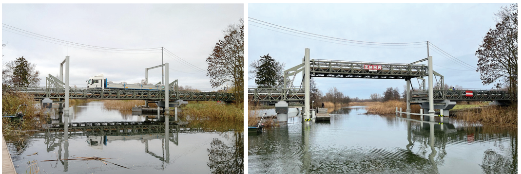
Figure 13. Views on the bridge over the Tuga River in Żelichowo, Poland: A road and sailing serviceability stage
