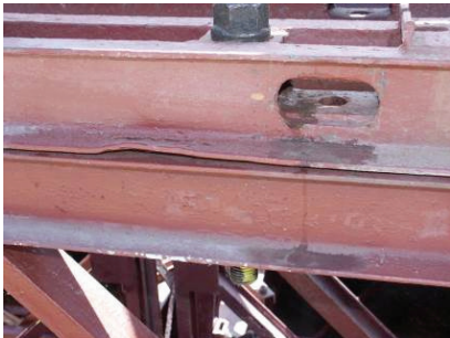
Figure 8. Bridge MS 22-80 type – deformations of panels examples on site
