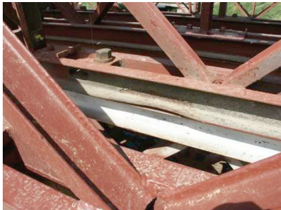
Figure 8. Bridge MS 22-80 type – deformations of panels examples on site
