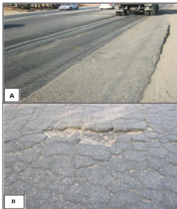
Fig. 2. (A) Rutting; (B) Fatigue cracking [16].
