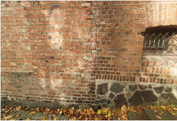
Photo. 2: No masonry bond at the junction of the former office spaces (A) with the former staff apartment (B), part of which are the rooms of the Southern Guardhouse
