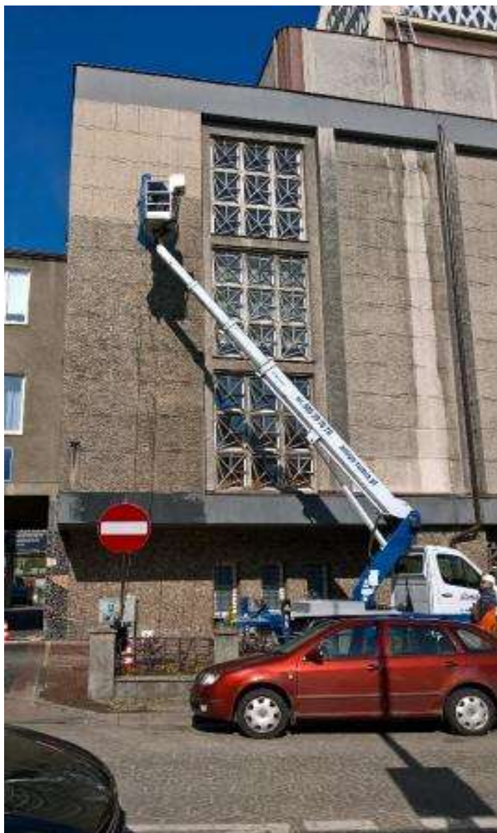
Photo 17. Comparison of the structure and color of the facade a) before and b) after its cleaning - on the example of the eastern facade (from the side of Monsignore Hilarego Jastaka Street) (street names as of 2023) (photo by Jacek Bramorski)
