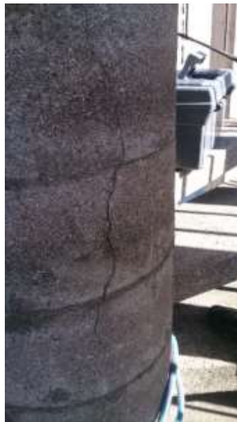
Photo 5. Outlined, in the line of the axial anchorage, prefabricated steps of the spiral stairs leading to the top of the belfry tower (photo by Maciej Niedostatkiewicz)
