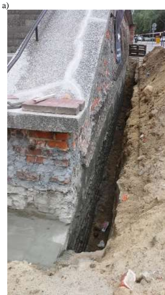
Photo 14. The wall at the entrance from the west elevation (along 3 Maja Street) during renovation works: a) dismantled cracked stone cladding and implementation of vertical damp-proof insulation, b) repaired cracks in the terrazzo cladding of the wall cap (names of the street as of 2023) (photo by Jacek Bramorski)
