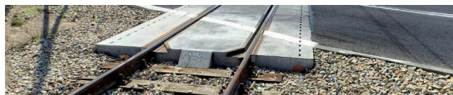
Fig. 8. Concrete level crossing slabs
