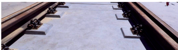
Fig. 7. Module of the level crossing during construction
