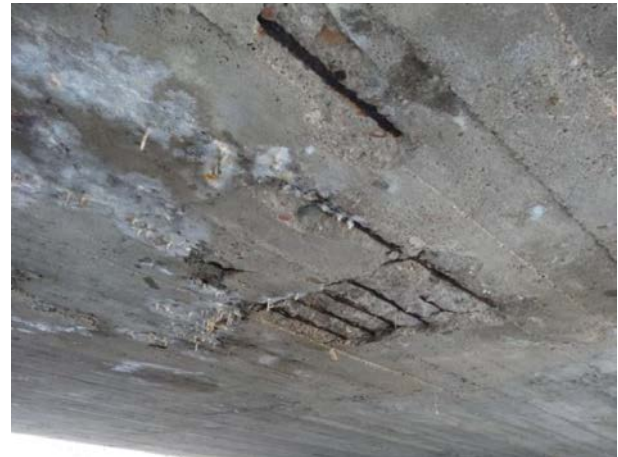
Figure 3. Bottom of the slab
