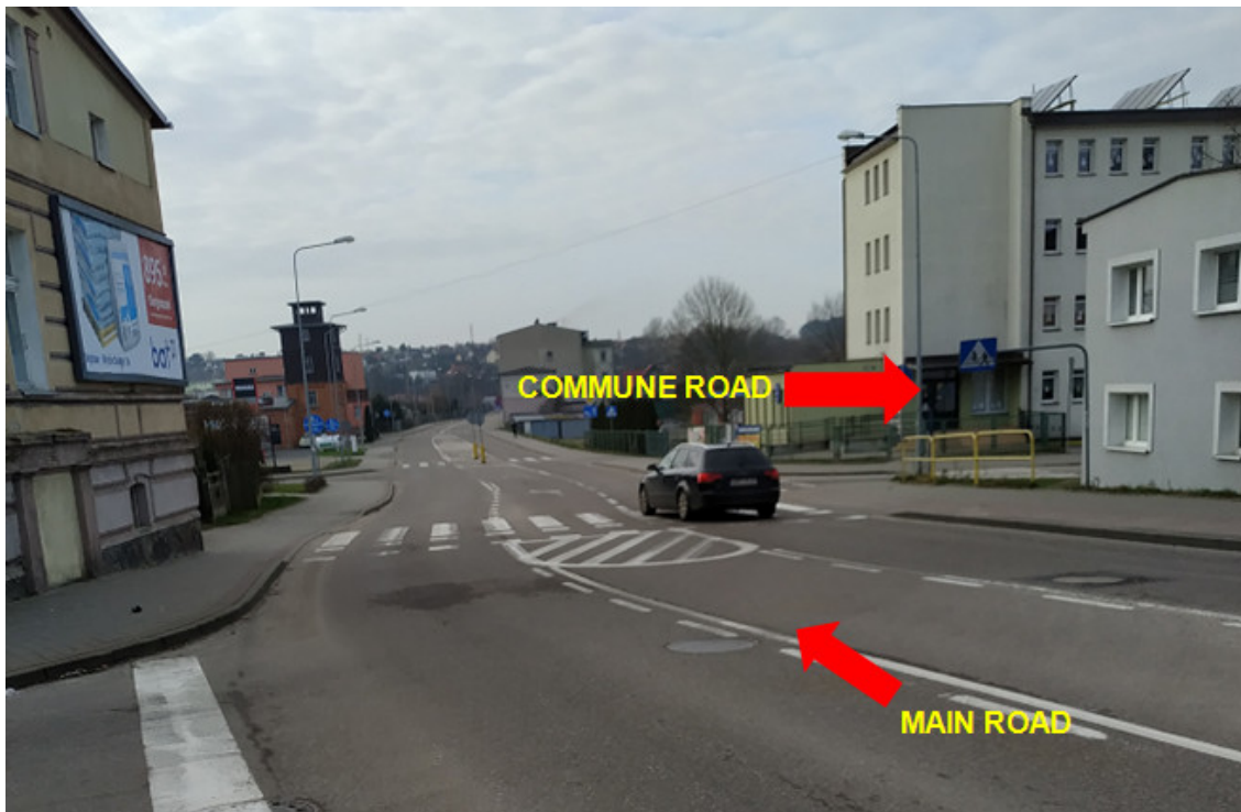
Figure 2. View of the intersection of the main road with the commune road.
