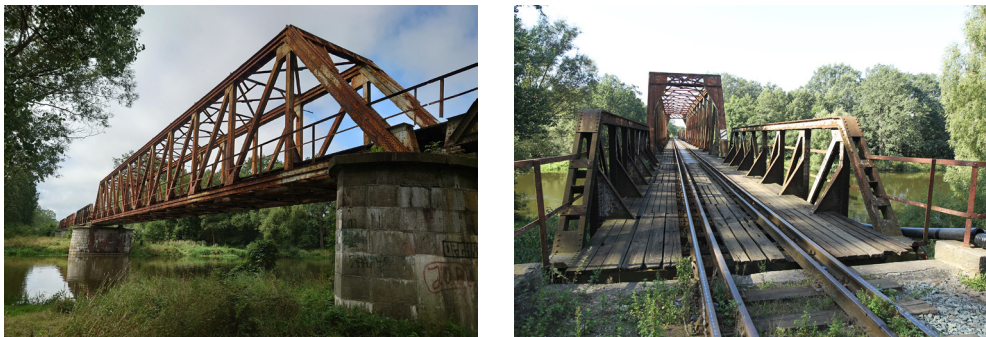
Figure 1. View on railway truss bridge
