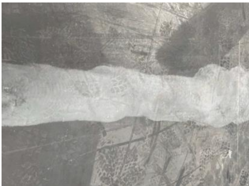
Fig. 6. Concrete industrial floor (Example 1) during repair: making an addition to the basin formed after the removal of the process channel [38]
