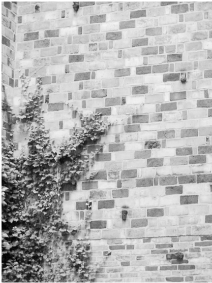
Photo 1. Clinker façade – Helmholtzstrasse multifamily house Source: B. Macikowski (photos. 1-11).
