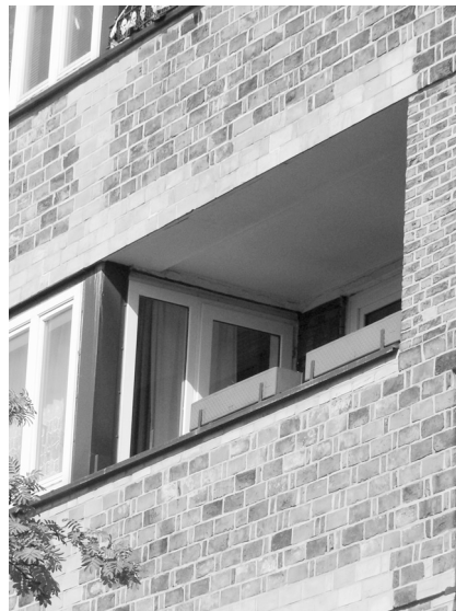
Photo 9. „Lunapark” multifamily complex – detail
