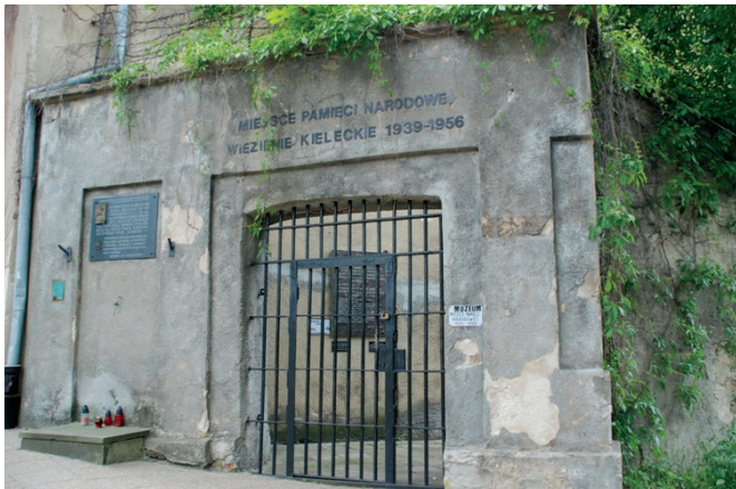
Fig. 5. Former prison in Kielce, a main gate [27]
