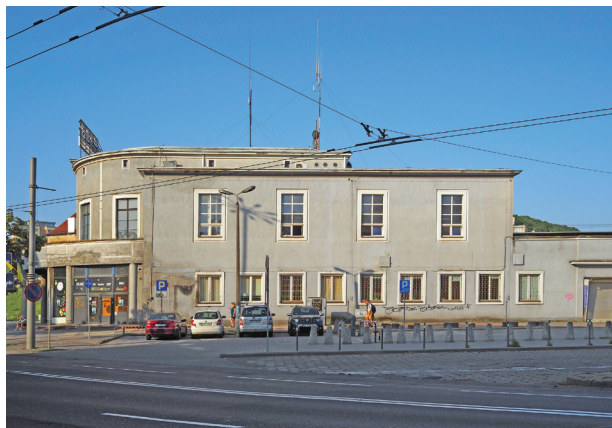
Fig. 5. Side elevation (north-east) of the Gdynia Główna Suburban Railway Station, June 2022 (before the start of conservation work).
