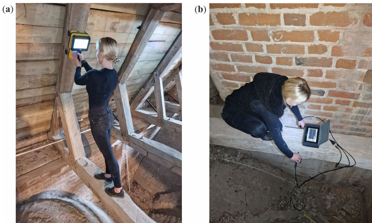
Fig. 3 NDT equipment used in in-situ tests: a ground penetrating radar b ultrasonic pulse velocity tester
