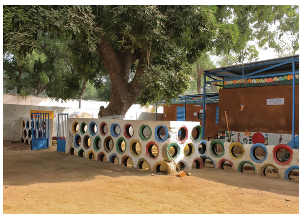
Fig. 4. Primary School, Quartier Dixième, Thiès, Senegal (source: image courtesy Let's build my school – humanitarian organization)
