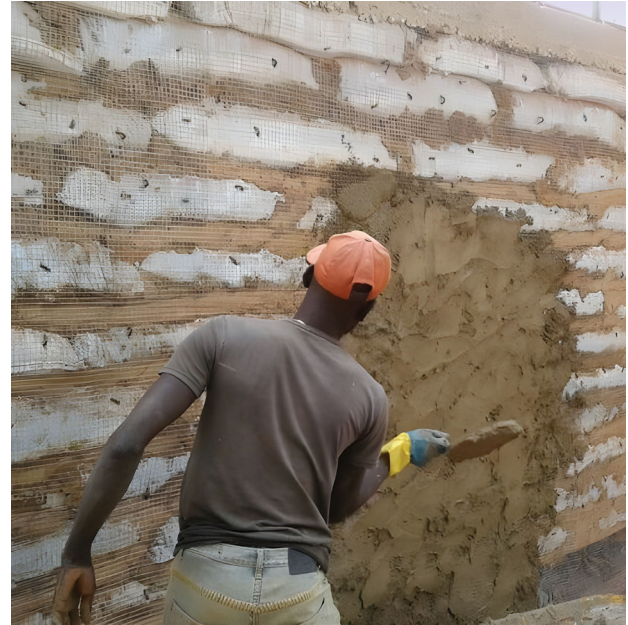
Fig. 6. Primary School, the Quartier Dixième, Thiès, Senegal. Sand and cement plaster (source: image courtesy Let's build my school – humanitarian organization)
